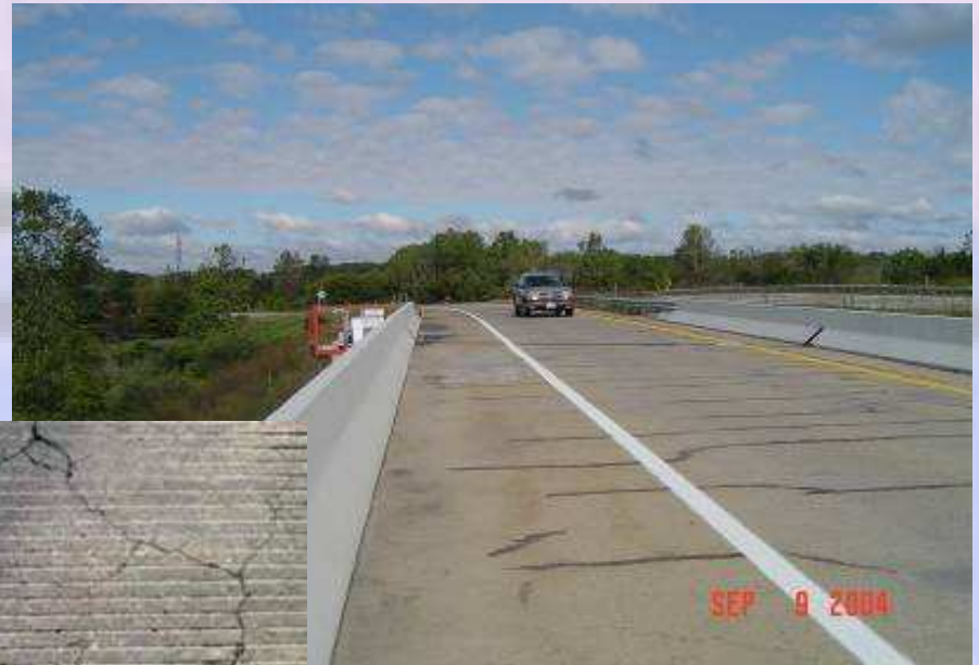
Crack Sealing
